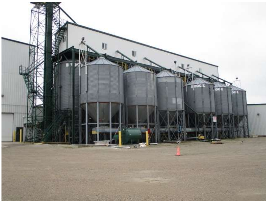
Commercial (galvanized) bulk hopper bottom storage bins – north of building #7
