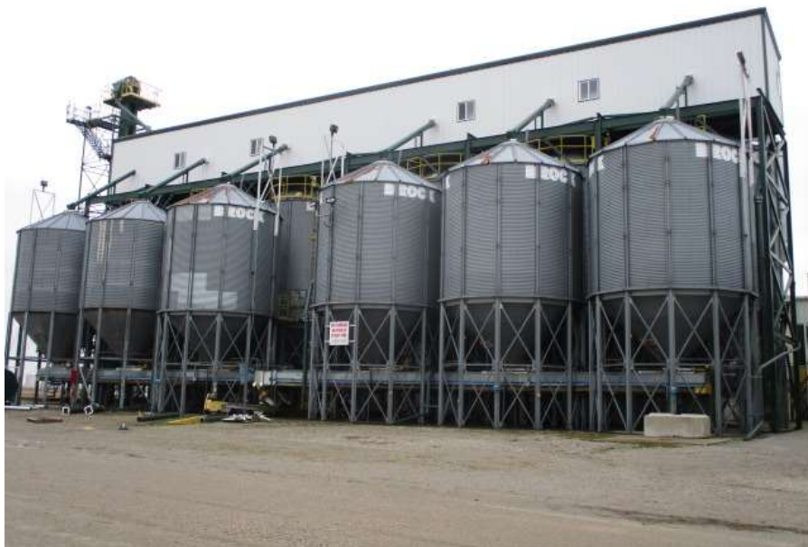
Commercial (galvanized) bulk hopper bottom storage bins – north of building #7
