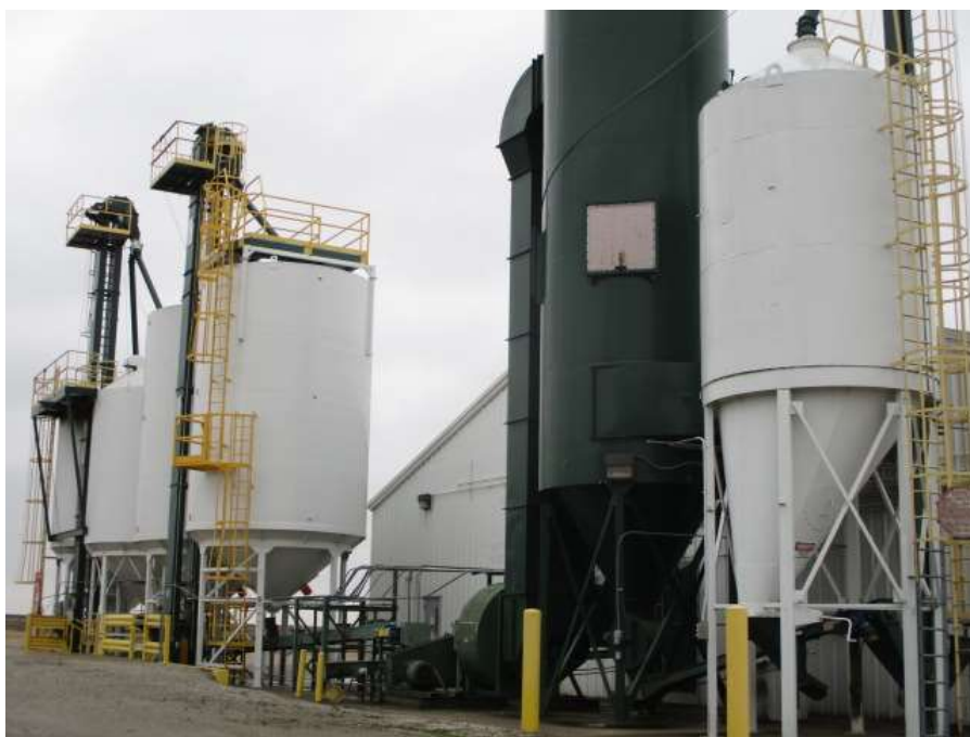
Freisen/Meridan hopper bottom storage bins – west of building #12
