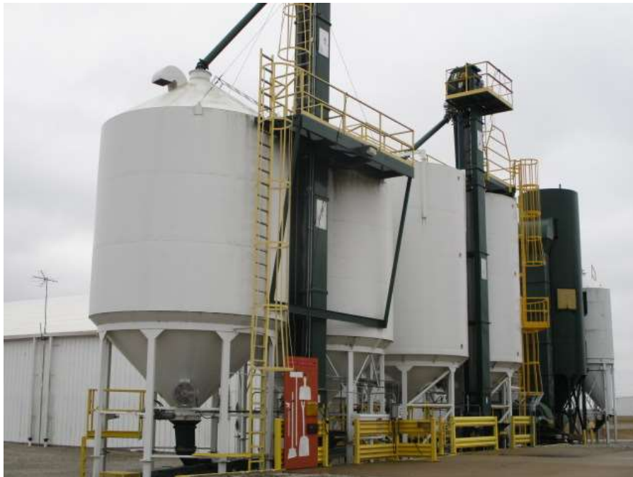
Freisen/Meridan hopper bottom storage bins – west of building #12
